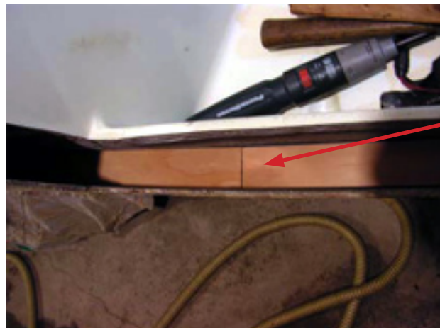
Staggered wood strip joint
