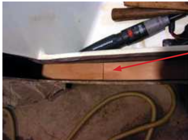
Staggered wood strip joint
